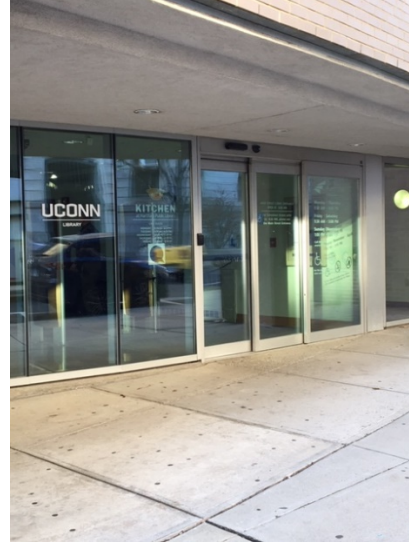
HPL side entrance off Arch St (2)
