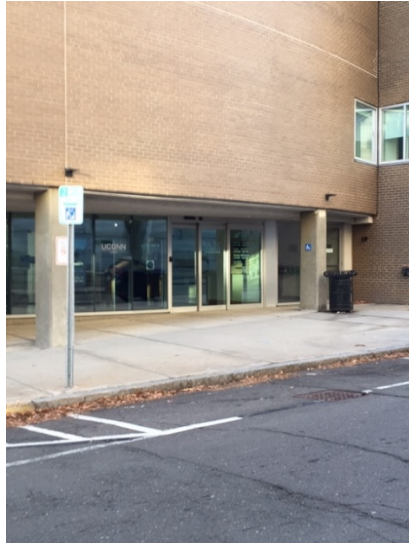
HPL Side entrance off Arch St (1)
