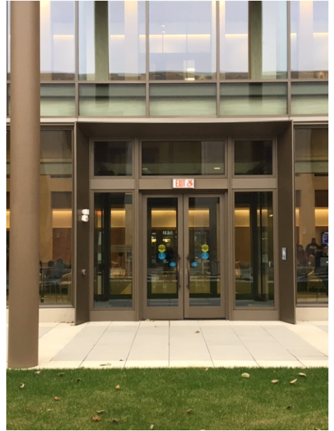
Courtyard building entry
