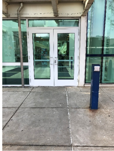
Accessible entrance on Franklin Street
