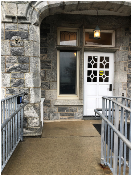
Accessible entrance on east side of building
