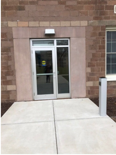
Accessible entrance on east side of building
